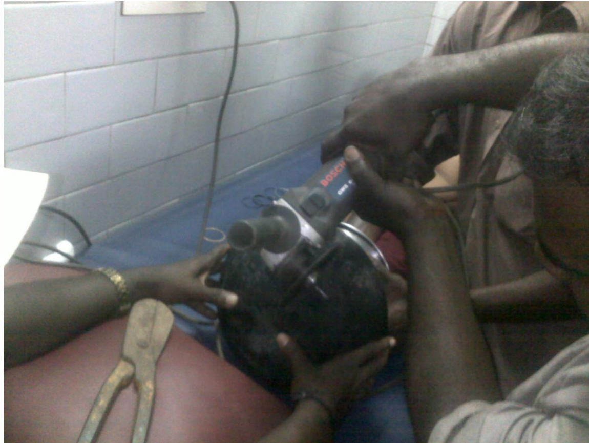
FIRST WELDER MAKES AN HOLE IN THE BASE
